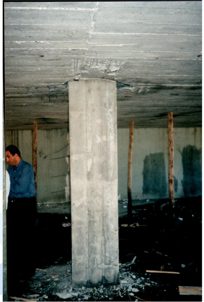
Figure 3. Punching damage under vertical loads
