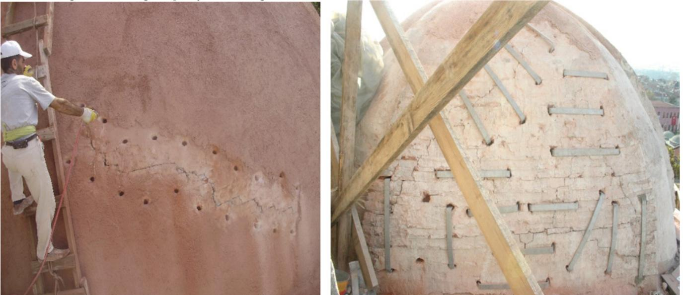
Figure 13. Cracks on corner dome at station 5 (left) damage on top of the pillar around the station 6 (right) [18, 19].
