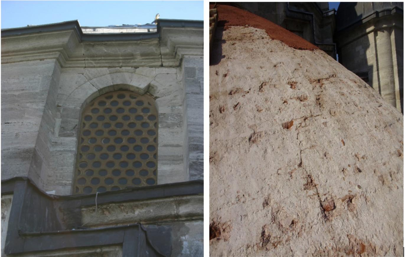
Figure 12. Damage around station 4 (left), failure cracks on the side dome at station 4 (right) [18, 19].
