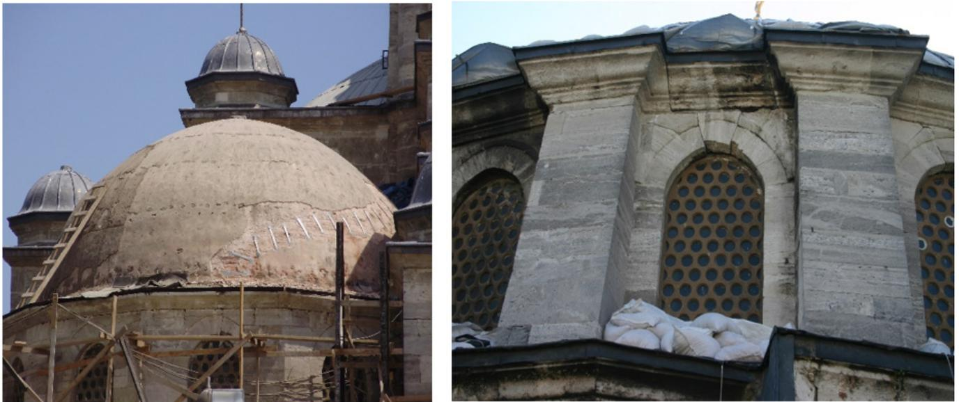
Figure 14. Dome damage at the corner around station 7 (left) serious damage at station 8 (right) [18, 19].
