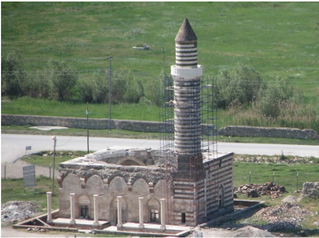
Figure 2. Damaged mosque after 2011 Van Earthquakes [19]
