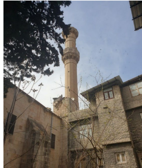
Figure 1. General view of the collapsed minaret from the rear courtyard after the earthquake
