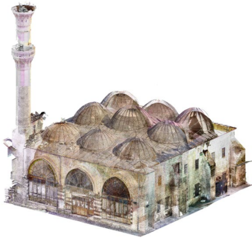
Figure 4. External view of the mosque and minaret point cloud model after the earthquake and Pazarcık earthquake east direction
