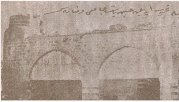
Figure 2. View of the dome and minaret destroyed by the French in 1920
