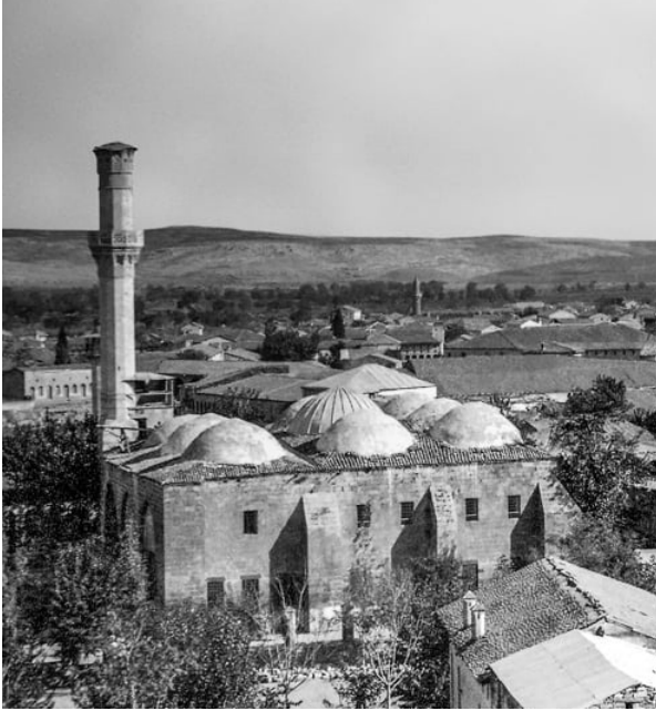
Figure 3. View of the reconstructed minaret with a single balcony
