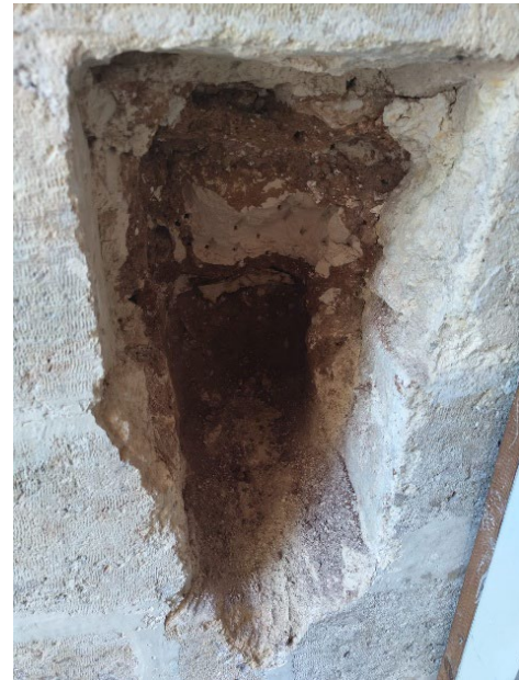
Figure 6. View of the irregular rubble fill inside the pulpit
