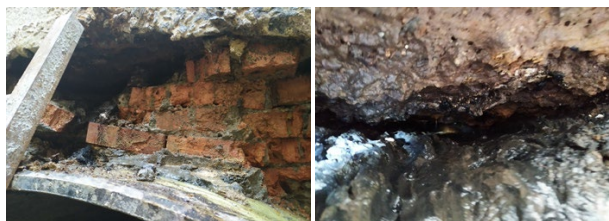
Figure 2. Photo of cavities in the upper part of the manifold above the fiberglass pipe
