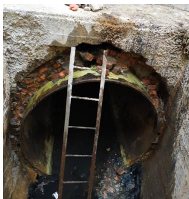
Figure 1. Junction of fiberglass pipes to the outer reinforced concrete structures of the chamber
