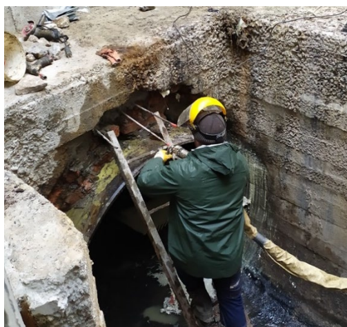
Figure 10. Injection process of polyurethane material SPT®
