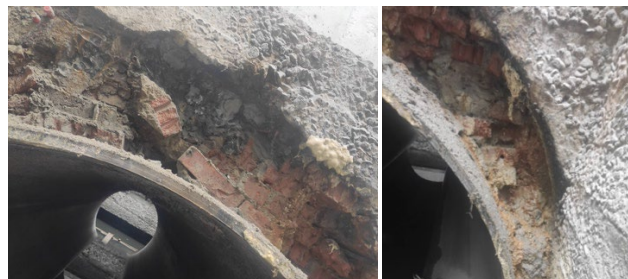
Figure 11. State of junction in 10 days after pressurizing
