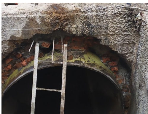
Figure 9. Mounting injection pipes and restoring damaged areas
