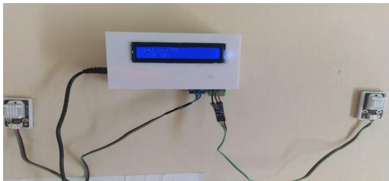
Figure 2. Installation of Automated Sensor for collecting data
