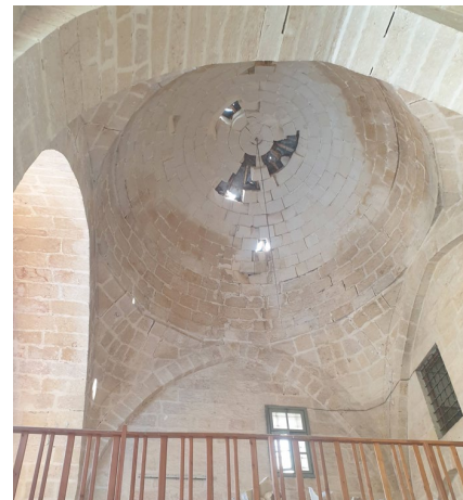
Figure 3. Dome damage
